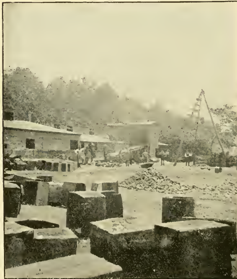
The Old Foundry—Rear View.
